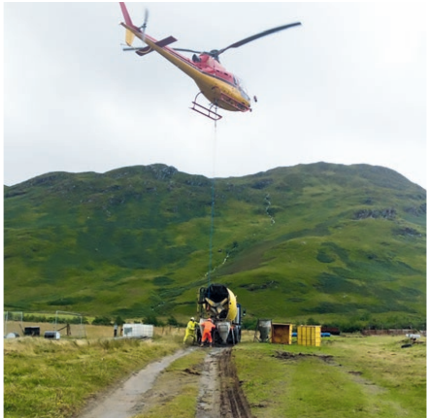
A helicopter lifts concrete to the Inverie dam project in a remote area of western Scotland.
