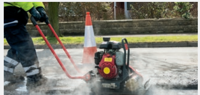
Large and small surfacing projects
