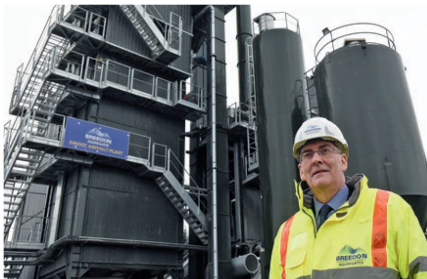
The new asphalt plant at Daviot, near Inverness, commissioned at the beginning of 2016.
