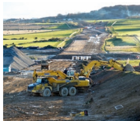
Under construction: the Aberdeen Western Peripheral Route.
