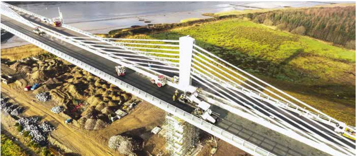
Above: The Rose Fitzgerald Kennedy Bridge, the longest in Ireland, part of the New Ross Bypass in County Wexford
